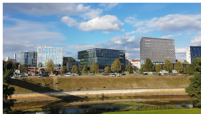
Fig. 2. New Business Centre on the embankment of river Nemunas, Kaunas (photo taken by Vytautas Petrušonis, 2020).
