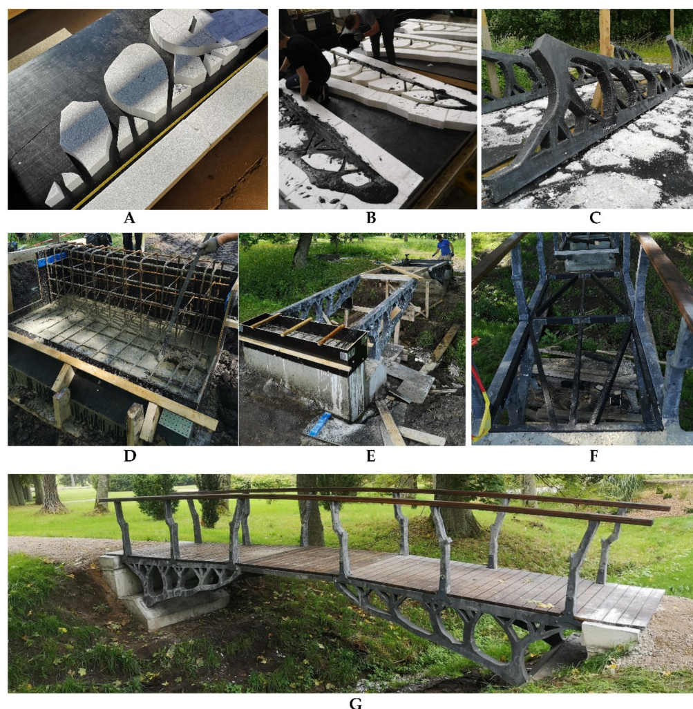
Figure 7. The construction of a prototype footbridge: (A) preparation of formwork; (B) pouring UHPC mix; (C) demolding UHPC trusses; (D) construction of foundation; (E) installation of UHPC trusses; (F) trusses connected with braced timber frame; (G) finished prototype bridge.
