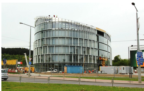
Fig. 1. An original office building, Vilnius
