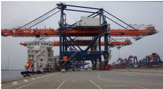
Fig. 1. Container crane in port of Rotherdam
