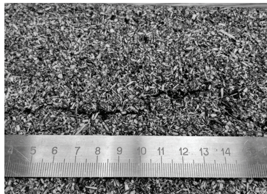
Fig. 11. Cracks which formed on the composite surface during hardening process, when the 0/2.5mm fraction was used
