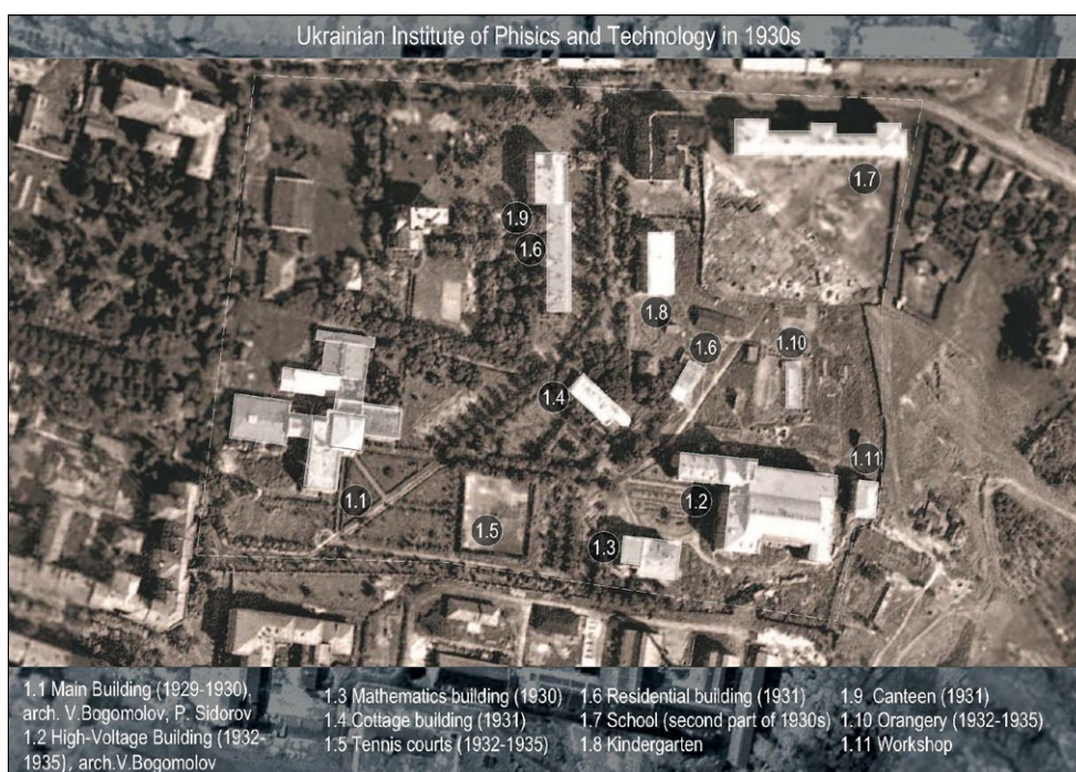
Fig. 1. UIPT complex scheme as in the 1930s; by K. Didenko based on a 1941 German aerial photo
