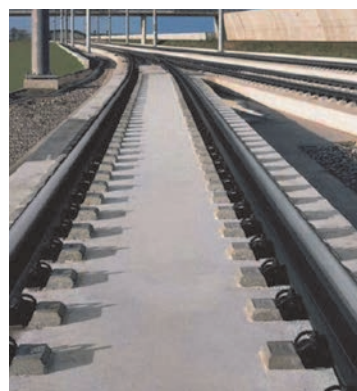
Figure 4. Slab track structure "Rheda 2000"
