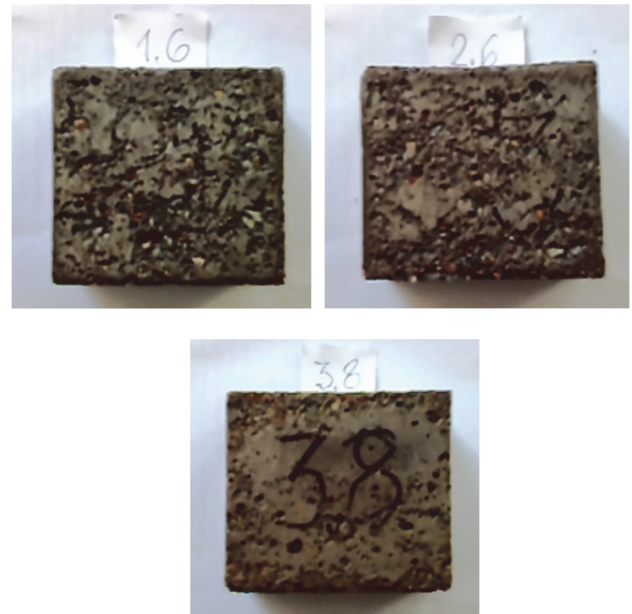
Fig. 9. Destruction surface of samples with different cements after 21 cycles of freezing and thawing.
