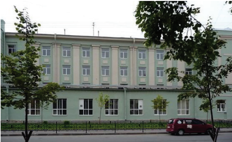
Fig. 11. Academic Gymnasium No. 56 in Saint Petersburg, designed by Trotsky and Martynov, 1936 [24].
