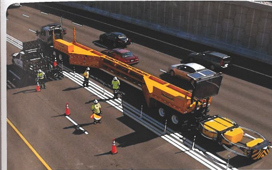
Illustration 6 - Mobile barrier in road work zone © www.mobilebarriers.com
