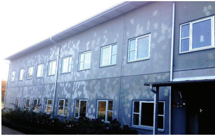
Fig.13. Facade in Helsingborg during repair
