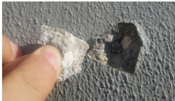
Fig.3. Maximum size of scales- about 30mm
