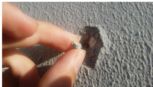
Fig.4. Maximum size of reacted aggregate- 4-5mm
