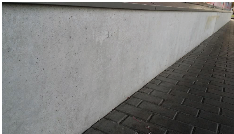
Fig.14. No AAR found on socle elements in Kaunas
