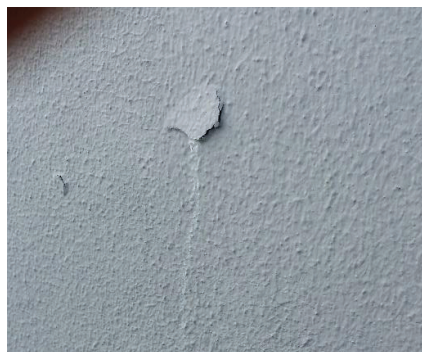
Fig.12. Reaction products leaching from the scales
