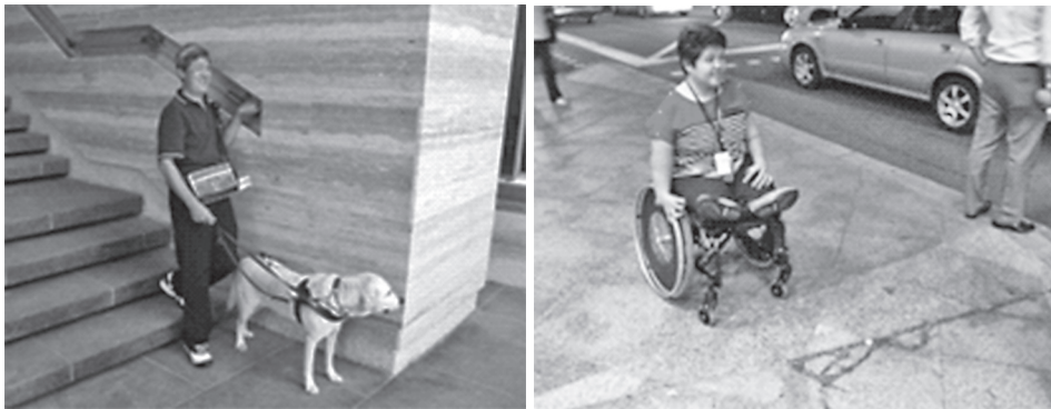
Fig. 15. The confusingly overdesigned handrail is too high to reach and does not serve its real function (a). Accessible travel route has sudden level changes (b) (photo by G. Stauskis)
