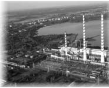
Fig. 6. Lithuanian Power Plant
