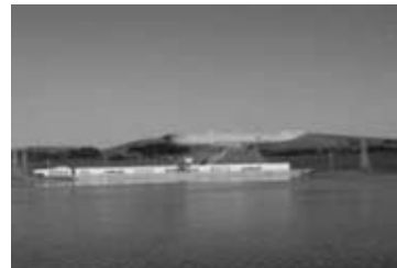
Fig. 4. Kruonis Pumped-storage Hydroelectric Power Plant
