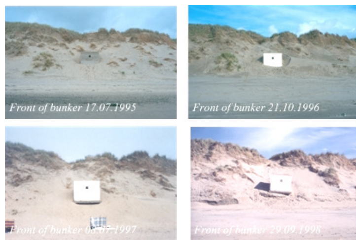
Fig. 3a. View directly in front of the war bunker. In 1995, a Second World War bunker became visible in the foredunes and provided a new fixed point. Observe the deflation of sand
