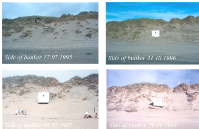
Fig. 3b. View from the south side of the bunker. Observe the exposure of the south-facing window and undercutting of the concrete platform
