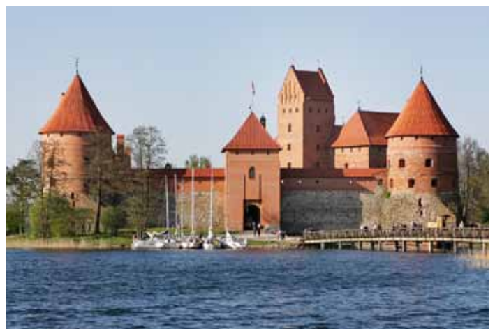
Fig. 6–8. Trakai island castle: the ruins of the castle palace in 1939; the restored palace in the castle (2012); the view of the entirely restored castle (2012).
