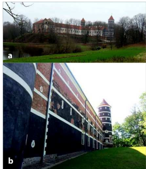
Fig. 10. Restored western wing with north and south-west towers of Vytėnai castle: a - 2012, b - 2013. Source: Genytė, 2012, 2013
