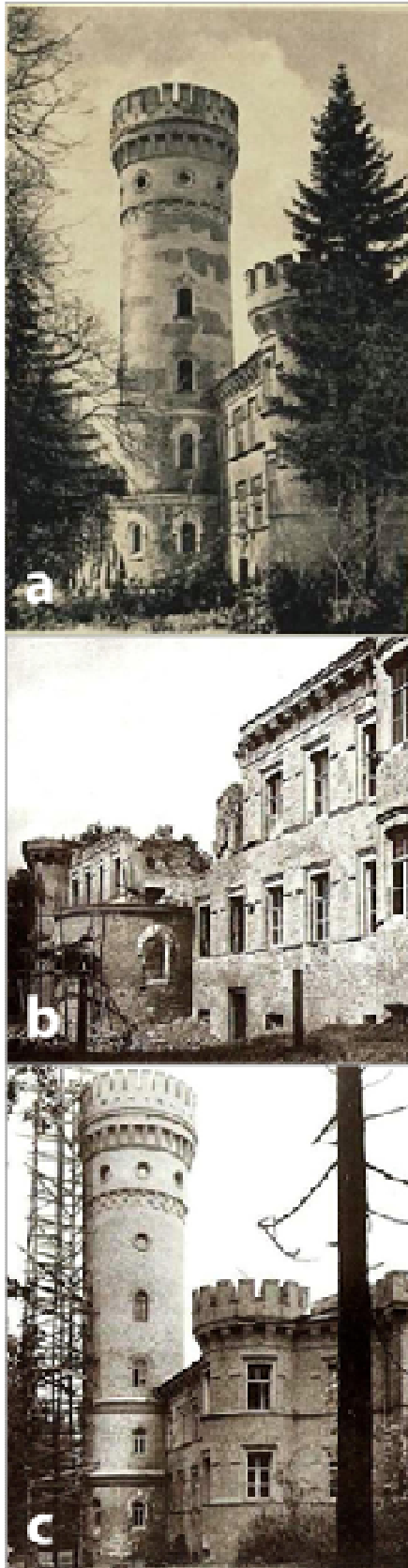
Fig. 7. Grand Tower and the South building restoration of Raudonė castle: a - 1941, b - situation after the Second World War, c - situation at the ending of reconstruction in 1968. Source: Vilnius County Archives
