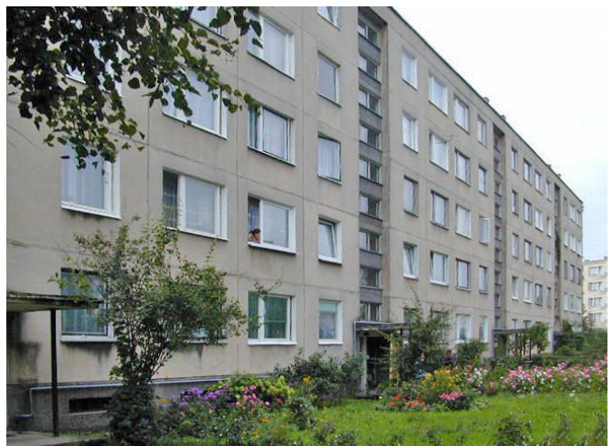
Fig. 2. The existing 5-storey prefabricated panel housing block of 30 apartments at Architektų Str. 212 in “Lazdynai” residential area (Vilnius) is planned to be renovated. The original project from 1970 (a); the present view, 2011 (b).
