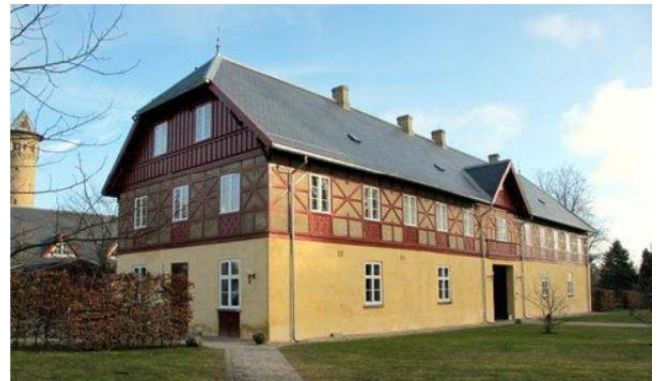
Fig. 5. Kavalergården building after refurbishment
