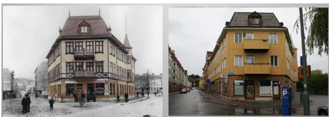
Fig. 3. Example of refurbished building when energy performance was increased to meet modern standards, but the authentic look of the building was destroyed.
