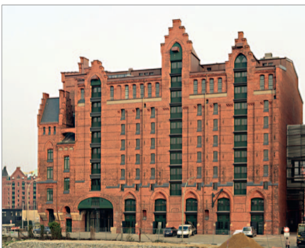
Fig. 9. Historic building reconstruction in Hamburg
