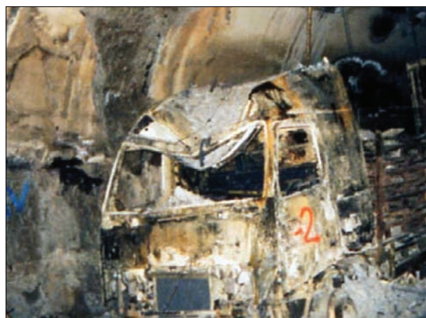
Fig 1. A vehicle after fire in the tunnel
