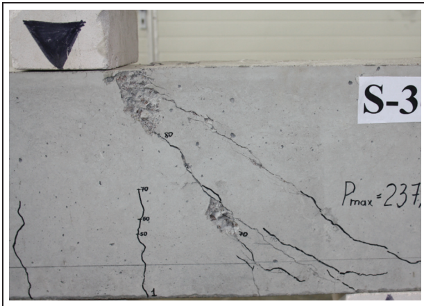
Figure 7. Cracking pattern at failure for the test specimens
