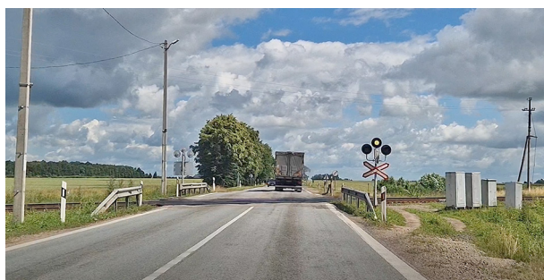
Figure 5. A railway crossing at 42.450 km of the A12 road
