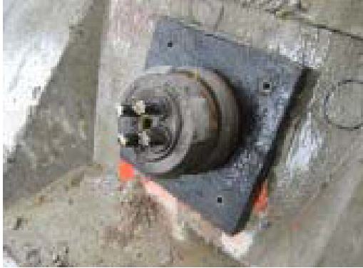
Fig. 4. Standard anchor (Rotar 2009)
