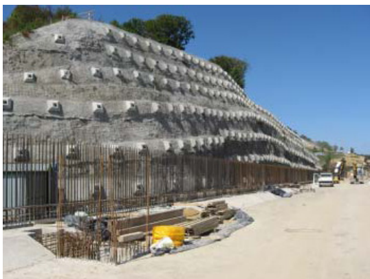
Fig. 5. Testing field for prestressed geotechnical (Rotar 2009)
