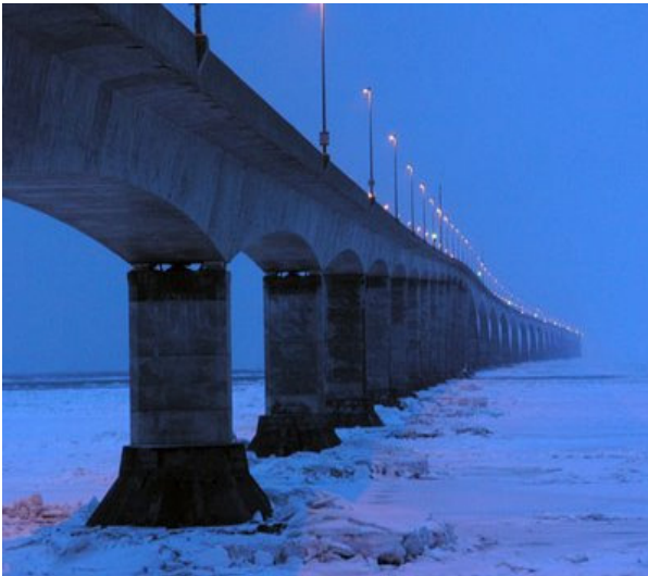
Fig. 7: Innovative design of bridge piers ( www.confederationbridge.com )
