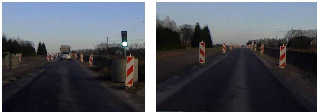
Figure 1. Work zone traffic management and driving conditions
