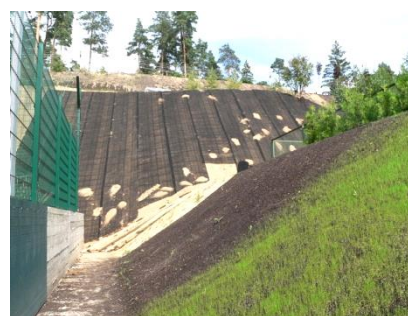
Figure 9. Reinforcement of embankments by road grids
