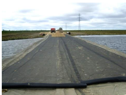
Figure 8. Application of basalt grids in road construction
