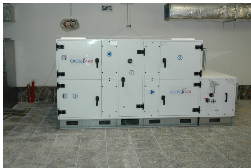
Fig. 1. AHU with EC motors
