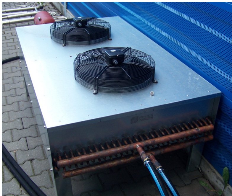
Fig. 2. Dry cooler used in the experiment
