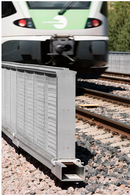
Figure 1. Low-height noise barrier (Sound Im, 2019)
