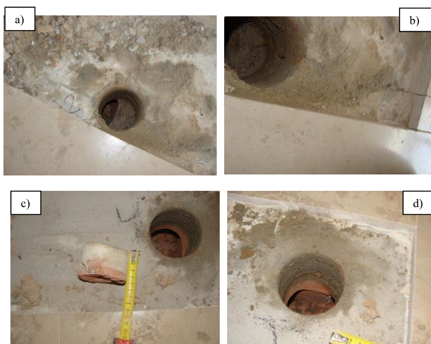
Figure 1. Examples of opencast works from floor layers: a, b) no. 2, c, d) no. 4
