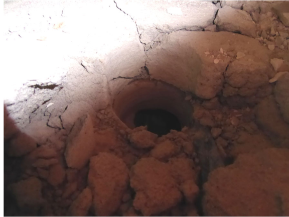
Figure 3. View of floor layers during demolition works
