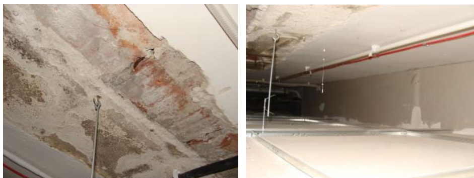
Figure 2. Views of the construction of Ackerman floor from the bottom
