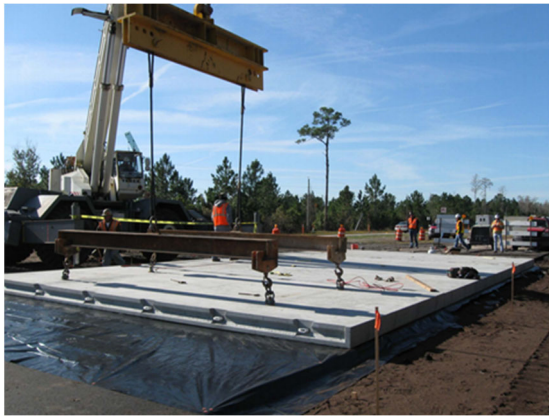
a) PPCP continuous construction
