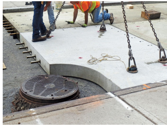
b) JCP continuous construction
