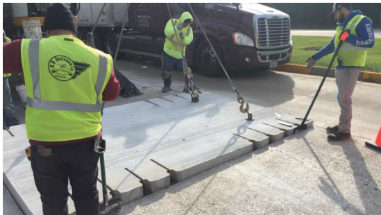
c) JCP intermittent repair
