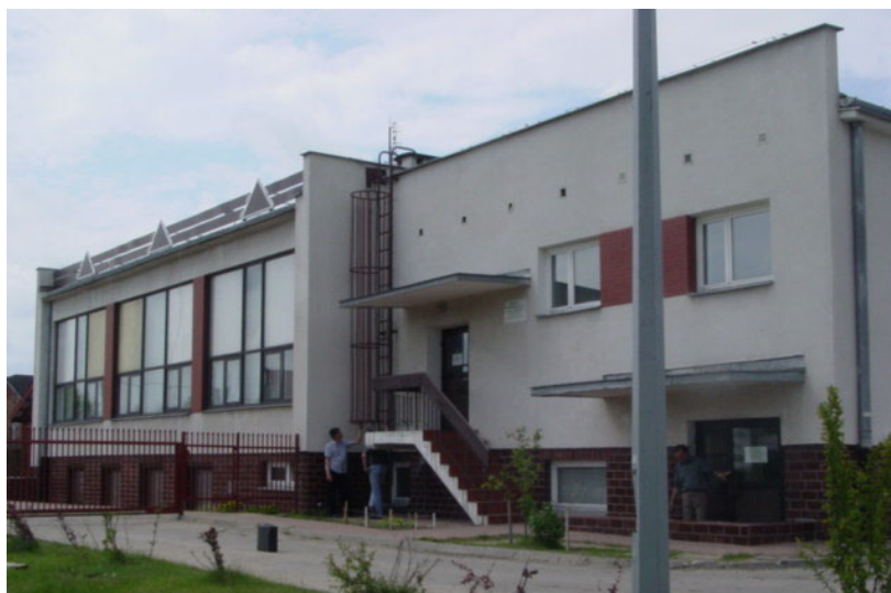
Figure 1. Building of the indoor pool
