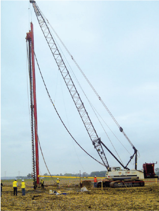
Fig. 1. Installation of ACIP Piles by fly-drilling technique
