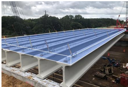
Fig. 1.13. Layered precast concrete girder–concrete deck structural system
