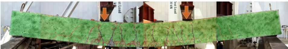
Fig. 3.26. Cracking pattern of slab S-2
