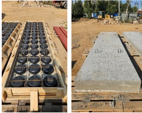
Fig. 3.21. Construction process of layered concrete slabs
