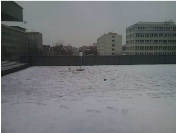
Fig 2. Placement of the rain gauge on the roof of the building of Library of the Technical University in Košice
