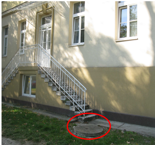
Fig 4. Percolation shaft in the area of the Technical University in Košice
