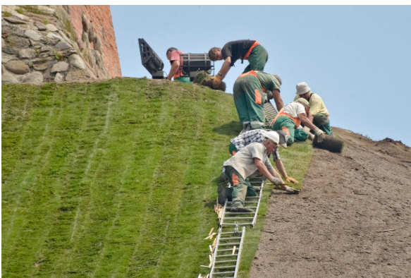
Figure 15. Three-year-old turf installation on Gediminas Hill slopes view in 2013 (D. Umbrasas photograph)
