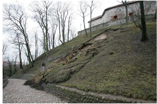
Figure 10. Gediminas Hill landslide in 2008 (V. Balkūnas photograph)
