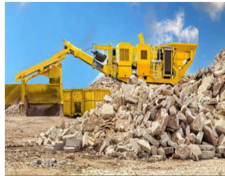
Figure 1. Selective demolition and sorting of construction and demolition waste
