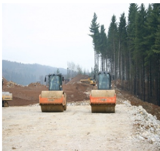
Fig 6. Two vibratory rollers (3.4.2009)
